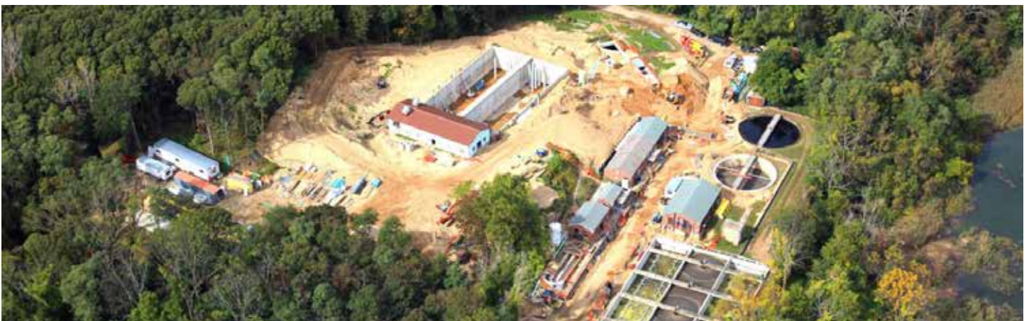
Photo of Kings Park Sewage Treatment Plant north of St. Johnland Road - County is illegally raising taxes & fees in Kings Park Sewer District 452% over 9 years after raiding approximately $200 million from sewer fund.
