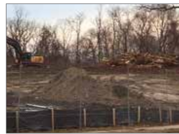
Construction of DEC office building resumes at park with conditions
